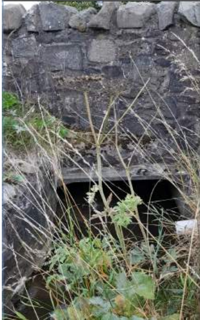
Photograph 4 - Upstream end of culvert at Dalmahoy Road
