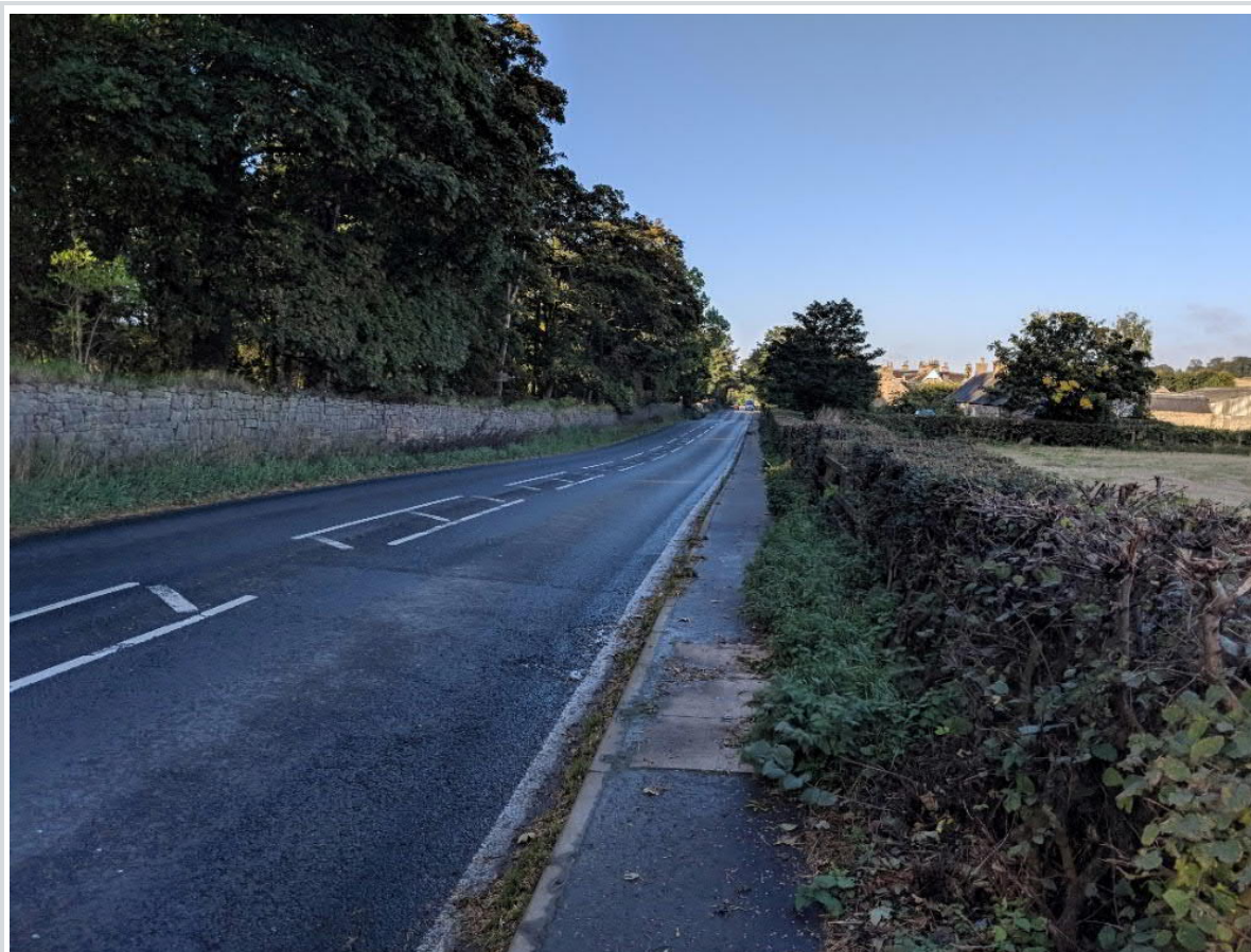
Figure 2.4: Footway on A71 (W)
