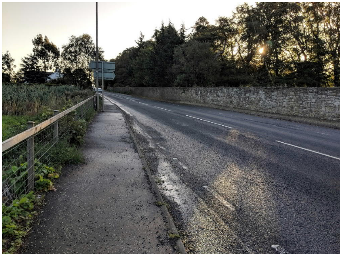
Figure 2.3: Footway on A71 (E)
