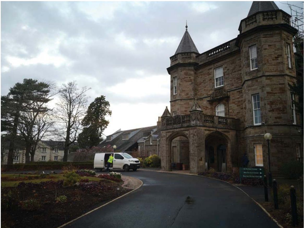
Plate 26: View north of Dalmahoy House, west entrance (Site 6)
