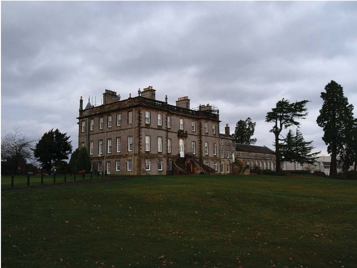
Plate 27: View northwest of Dalmahoy House, east entrance (Site 6)
